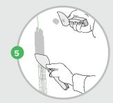
Also use joint paste or another filling material to conceal screw/nail heads. Allow the filler material to dry for 3 hours
